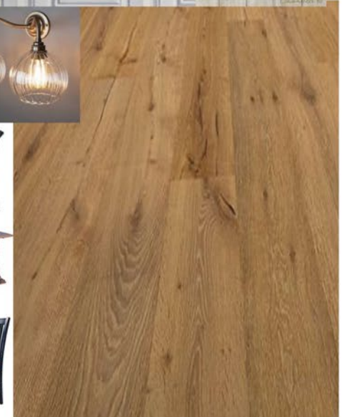
Existing timber floor
