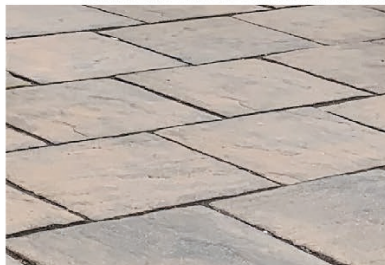
EXISTING PAVING JET WASHED AND RE-POINTED
