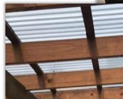
Existing pergola to be repaired with new clear polycarbonate roof.
