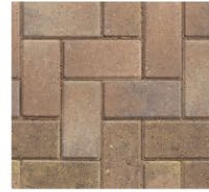
EXISTING BLOCK PAVING
